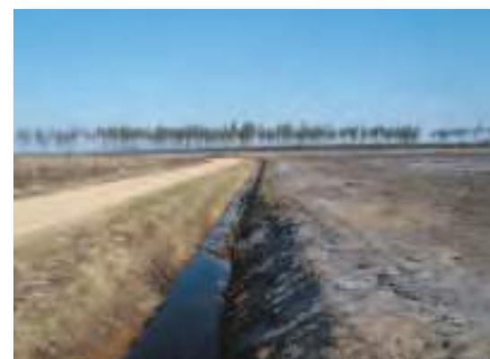
Site preparation with water distribution, Arengosse Demonstration site (R. Cordero Debets, EFIATLANTIC).
