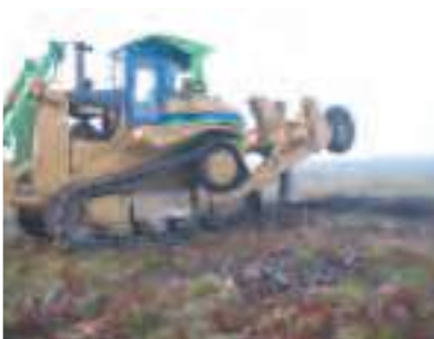
Subsoil site preparation, DS25 (R. Cordero Debets, EFIATLANTIC)
